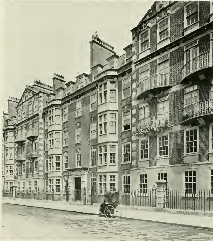
COLEHERNE COURT, OLD BROMPTON ROAD, LONDON. AN EXAMPLE OF EXTERIOR DESIGN, WITH PLEASANT WINDOWS OF A KIND NOT COMMON IN FLATS. THE BUILDING MATERIALS ARE RED BRICK WITH BATH AND PORTLAND STONE. THE RENTS, INCLUDING RATES AND TAXES, RUN FROM £130 TO £160 A YEAR
